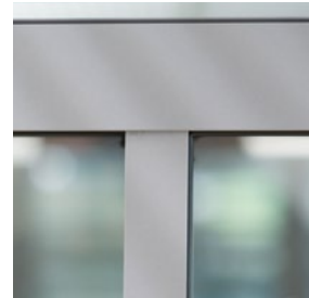
top-left: Exterior detail of frame: frame-lower transom
